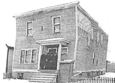
First Service Building, Concordia College, Edmonton, Alberta, 1926-1928. Concordia's first building
