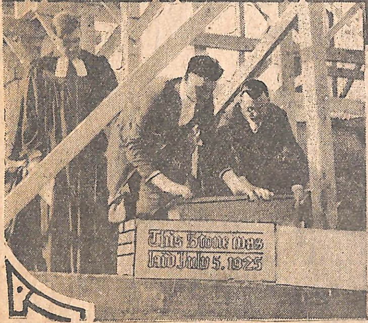
Above are scenes during the laying of the cornerstone for the fine Concordia Lutheran college, estimated to cost around $250,000, at the Highlands on Sunday afternoon. A portion of the crowd of 1000 spectators is seen in the top picture which was taken during the singing of the hymn, "A Mighty Fortress is Our God." In the lower picture are seen those charged with laying the cornerstone. On the right is G. H. Macdonald, architect, while in the centre is Rev. A. H. Schwermann, principal of the new college, and on the left is Rev. A. J. Muller of Calgary, president of the Alberta and British Columbia districts.
